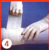
Apply Rapp-it around damaged area and tighten the wrap firmly
