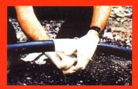
Rapp-it is roll of fibreglass bandage impregnated with water-activated resin which is ready to use once the foil pouch is opened. You simply immerse Rapp-it in water for 10 seconds, then apply by wrapping around the damaged area. A successful repair can be achieved in 30 minutes.
