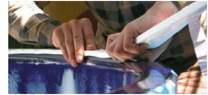
Installation of GORE® Gasket Tape Series 1000
